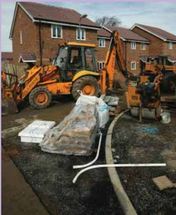
New Homes being built in the Thames Gateway
